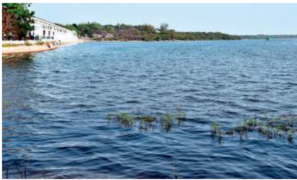
Though the water level at the Poondi reservoir is only one-third of its capacity, the Water Resources Department is not increasing the storage owing to work on shutters.
