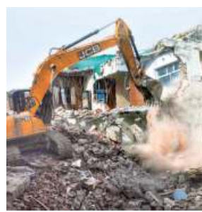
A house being demolished in Prayagraj. •PTI
