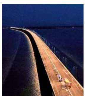
An aerial photograph of the Padma multipurpose bridge and railway project in Louhajang, Dhaka. •AFP
