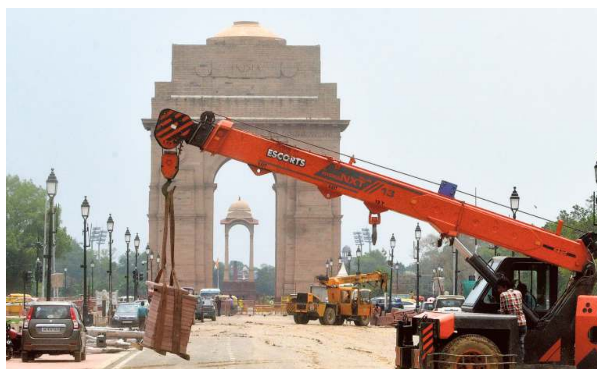
Almost ready: Construction work in full swing for the Central Vista redevelopment project near India Gate in New Delhi on Saturday. Central Vista Avenue is set to open in a few days. ■ R.V. MOORTHY
