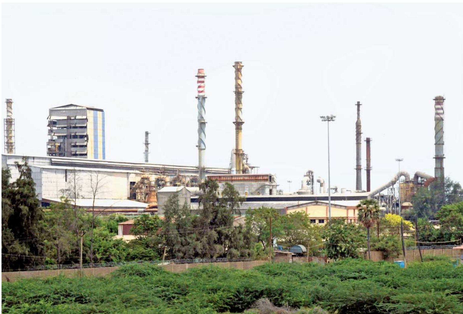
Under lock-down: A view of the Sterlite Copper plant in Thoothukudi. ■ RAJESH N
