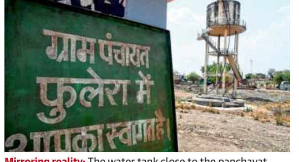
Mirroring reality: The water tank close to the panchayat office in the show is now a key poll plank. • A.M. FARUQUI
