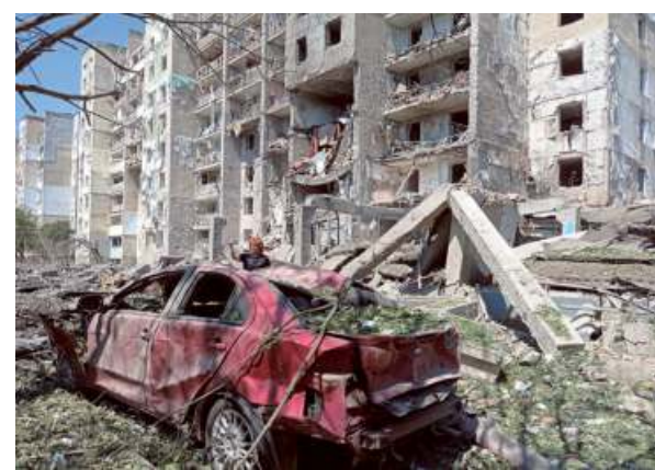
A residential building damaged by a Russian missile strike in Serhiivka, Odesa region, on Friday. ■ REUTERS
